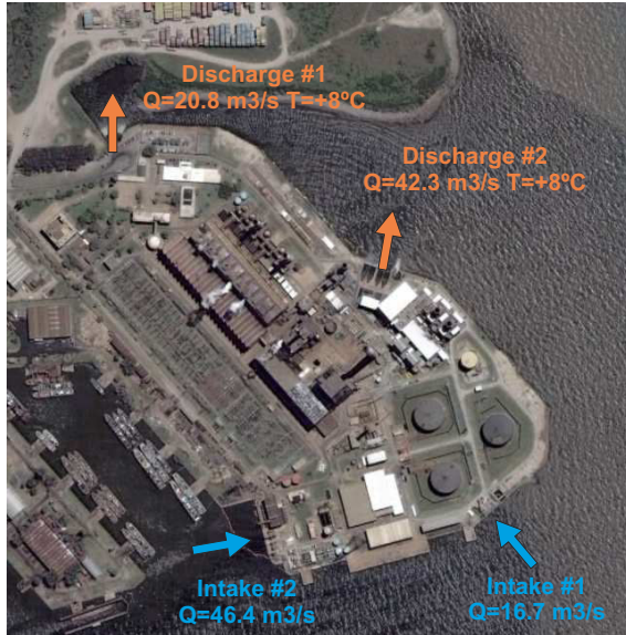
Figure 4. Discharges and intakes at Central Costanera.
